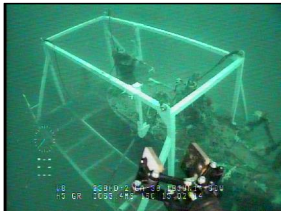
Figure 10 DSP in position. Taken on final flyover, shows CP connections in place with ROV grabber in foreground.
