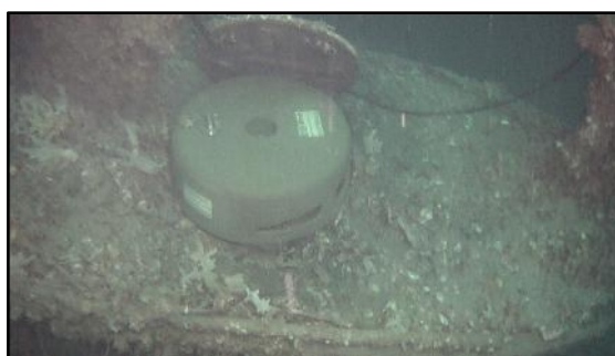
Figure 19 Hatch closure (Top Hat) in place, DSP removed. Anode connection cable visible
