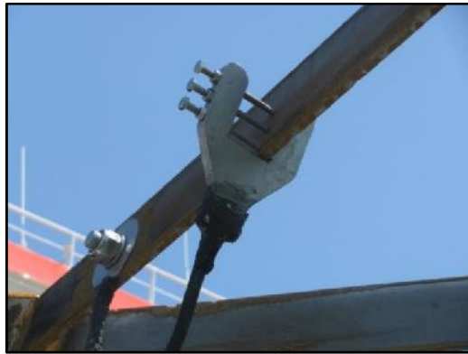
Figure 23 CPS Anode Pods; CPS Cable Connecting Clamp
